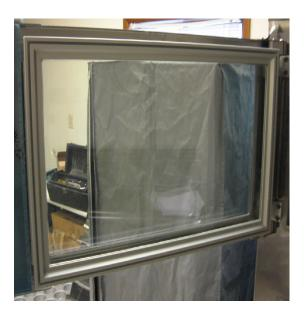
**Step 2** – We begin by removing the existing gasket from the door frame. The easiest way to do this is to pull the gasket out of the door frame. You can carefully take a flat headed screw driver in the corner of the door to help start the gasket. You want to make sure that you leave no gasket behind in the door frame.
